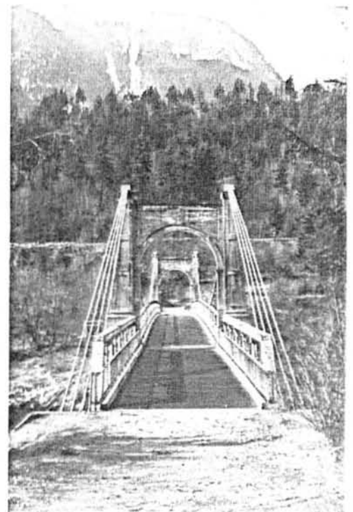
Suspension bridge from east bank
