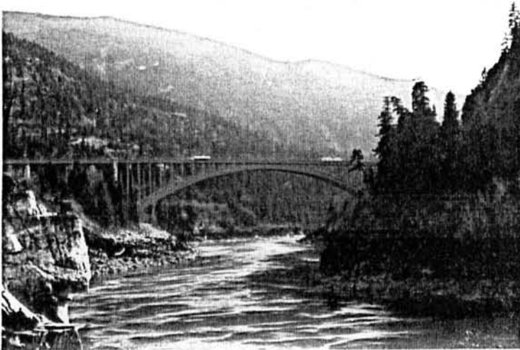
New Alexandra Bridge from viewpoint
